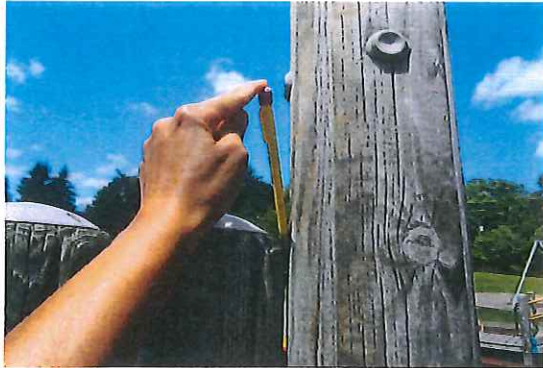
Climbing Wall - Eight drawstring entanglements at gaps in wood posts - CLASS A HAZARD
