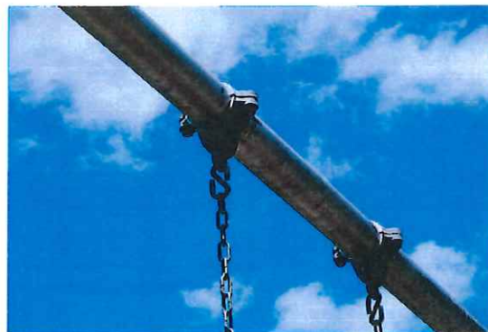
11ft. Swing Set - Eight "S" - Hooks starting to wear - MAINTENANCE
