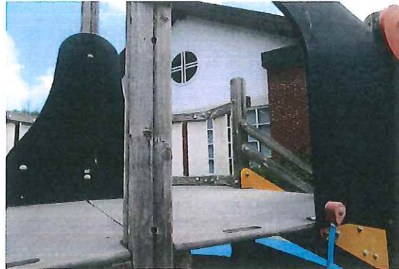
Pirate Ship - Wood worn, cracked & splintered - CLASS C HAZARD
