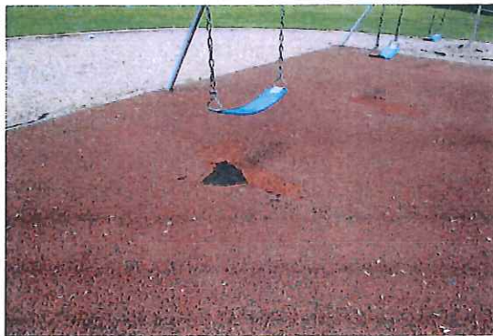
11ft. Swing Set - Surfacing is peeling - MAINTENANCE
