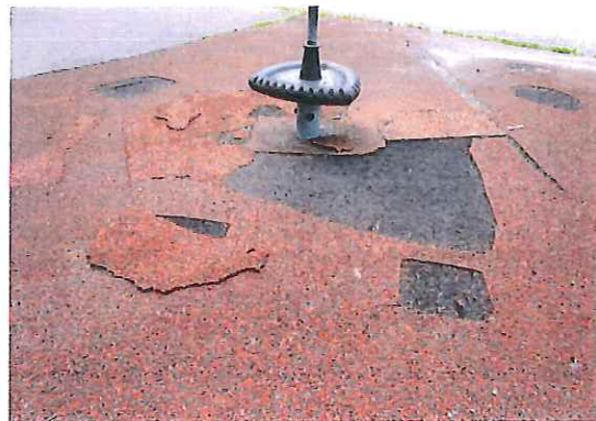
Spica GXY 8015 - Surfacing is peeling - MAINTENANCE
