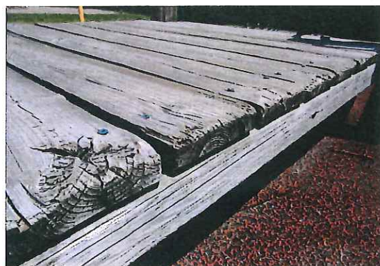
Mountain Climber - One cap missing - MAINTENANCE
