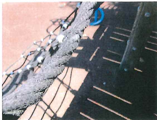
Transfer platform - Wood worn and splintered - MAINTENANCE
