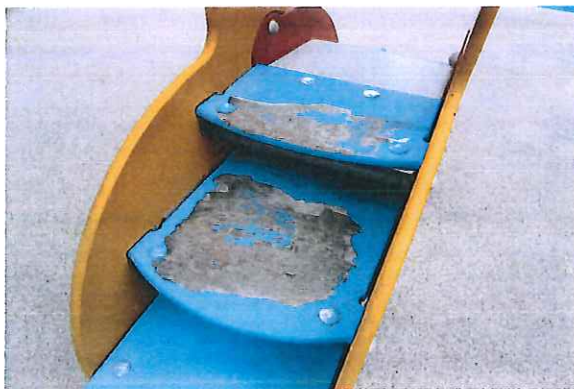
Mighty Musketeer (Kompan) - Wood splintered & paint peeling - MAINTENANCE
