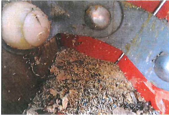
Pirate Ship - One cracked cap & insect damage - MAINTENANCE
