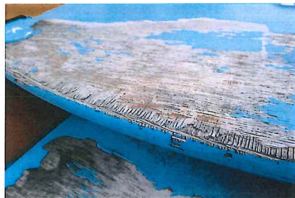
Mighty Musketeer (Kompan) - Wood splintered & paint peeling - MAINTENANCE
