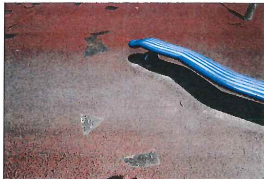
Argo GXY 8019 - Surfacing is peeling, missing & torn - CLASS B HAZARD
