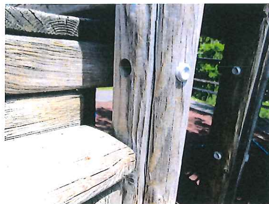
Mountain Climber - One cap missing - MAINTENANCE
