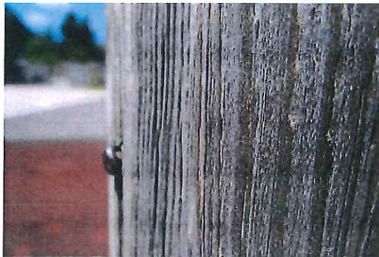
Climbing Wall - Screws exposed - CLASS C HAZARD
