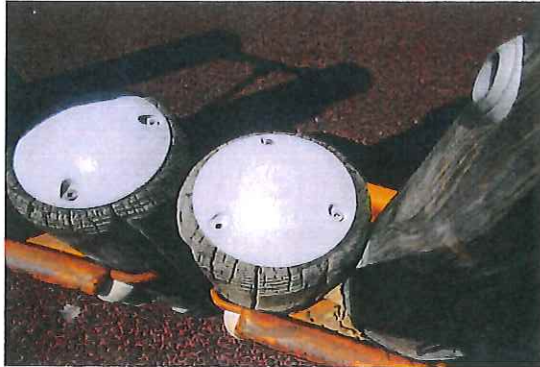
Climbing Wall - One bolt missing - MAINTENANCE
