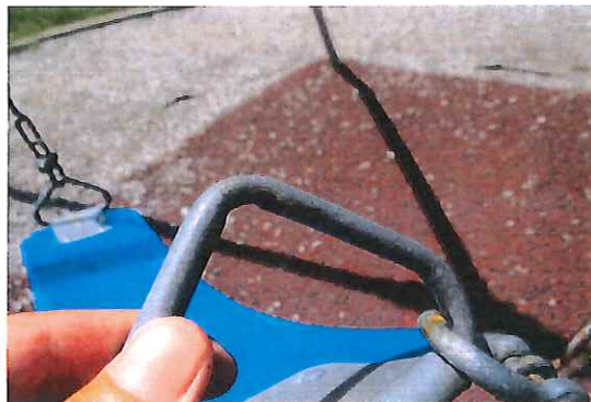
11ft. Swing Set - Eight "S" - Hooks starting to wear - MAINTENANCE
