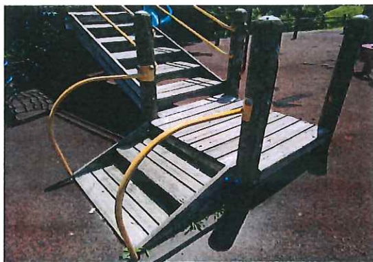
Transfer platform - Wood worn and splintered - MAINTENANCE
