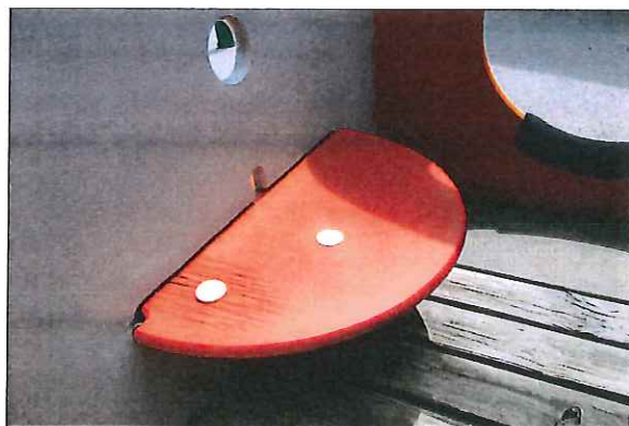
Labyrinth - Two seats loose - MAINTENANCE
