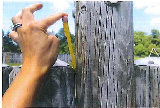
Climbing Wall - Eight drawstring entanglements at gaps in wood posts - CLASS A HAZARD
