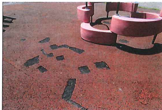
Argo GXY 8019 - Surfacing is peeling, missing & torn - CLASS B HAZARD
