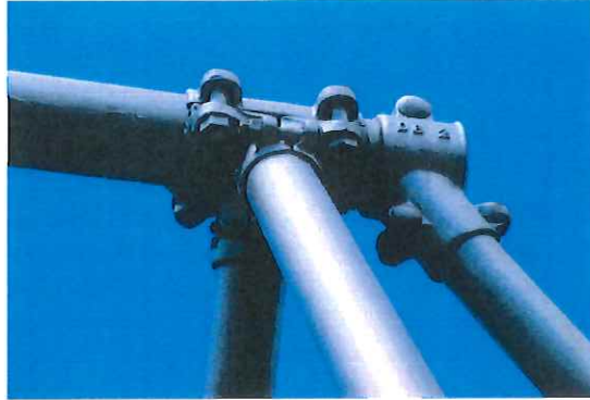
11ft. Swing Set - Four protruding bolts, drawstring entanglement at top hardware - CLASS A HAZARD
