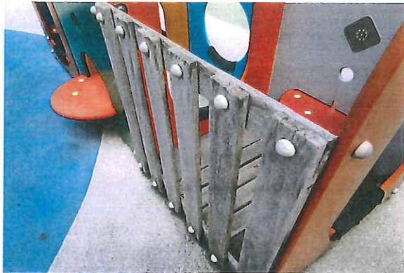
Labyrinth - Wood is cracking - MAINTENANCE
