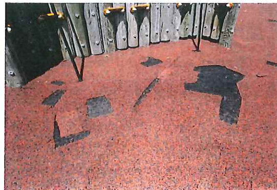
Structural Stability - Loose at Rope Bar posts - MAINTENANCE
