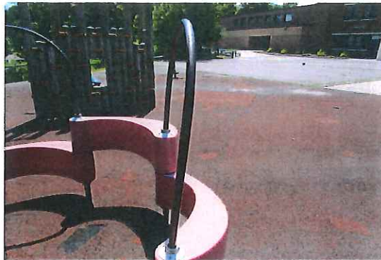
Playshell Climber -Surfacing areas peeling, torn & missing - CLASS B HAZARD
