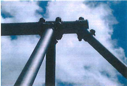
11ft. Swing Set - Four protruding bolts, drawstring entanglement at top hardware - CLASS A HAZARD
