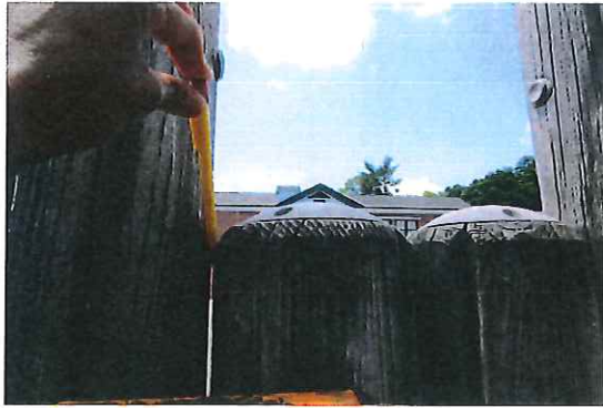
Climbing Wall - Screws exposed - CLASS C HAZARD
