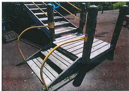
Transfer platform - Wood worn and splintered - MAINTENANCE
