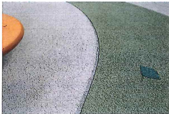
Daisy Springer - Surfacing is lumpy, seams separating - CLASS C HAZARD
