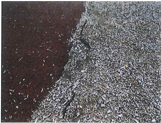
11ft. Swing Set - Use zone is inadequate at 3ft. On sides - CLASS C HAZARD
