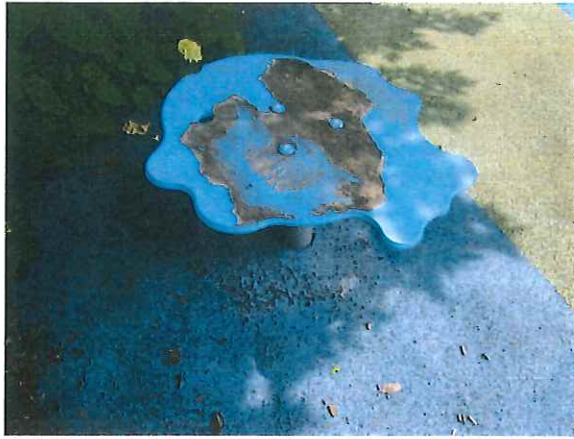
Play tables - Paint is peeling - MAINTENANCE
