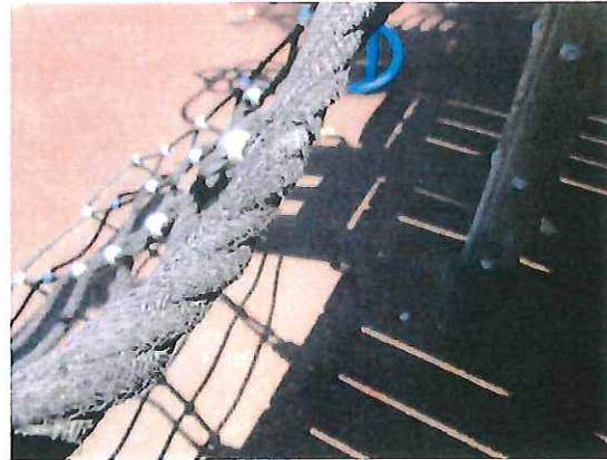
Transfer platform - Wood worn and splintered - MAINTENANCE
