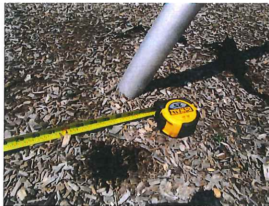
11ft. Swing Set - Use zone is inadequate at 3ft. On sides - CLASS C HAZARD
