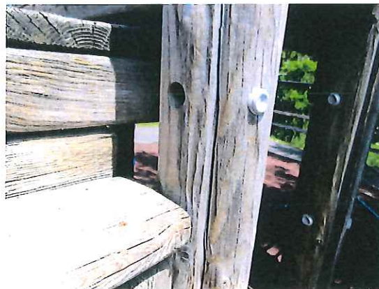
Mountain Climber - One cap missing - MAINTENANCE
