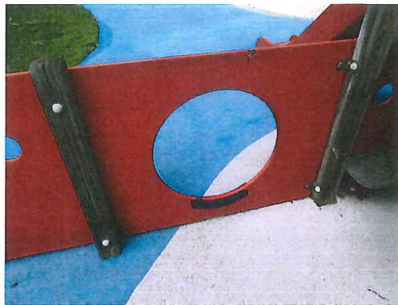
Pirate Ship - Crawl thru pad wearing & crack in crawl thru - MAINTENANCE
