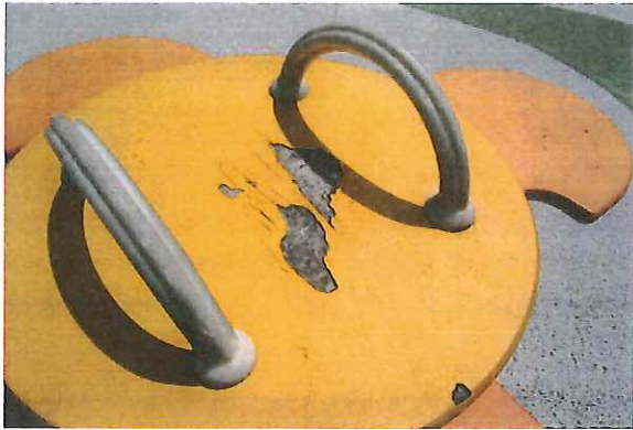
Daisy Springer - Surfacing is lumpy, seams separating - CLASS C HAZARD
