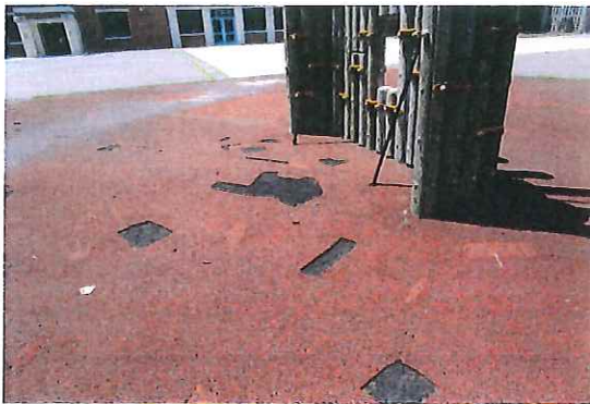
Structural Stability - Loose at Rope Bar posts - MAINTENANCE
