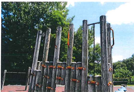
Structural Stability - Loose at Rope Bar posts - MAINTENANCE
