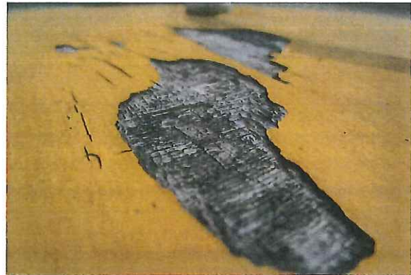
Daisy Springer - Surfacing is lumpy, seams separating - CLASS C HAZARD
